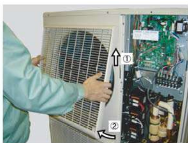
Remove the FAN GUARD by sliding upward.
