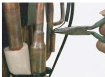
Remove the THERMISTOR SPRING.
