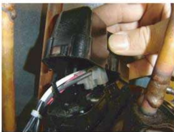
Remove the TERMINAL COVER.
