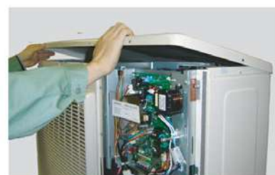
Remove the TOP PANEL.
