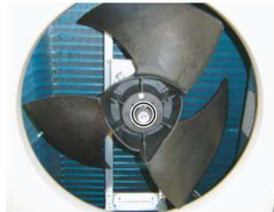
Remove the Hex Socket Screw. And remove the PROPELLER FAN. Note at the installation. Insert propeller Fan and Motor shall reference D cutting position. And the tightening torque at the installation. Tightening torque is from 10 to 15 N.M.
