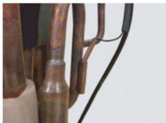
Remove the THERMISTOR.
