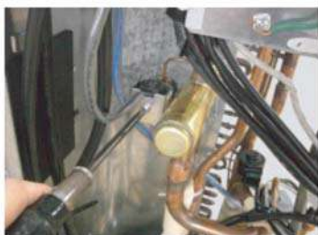
Remove the mounting screw.
