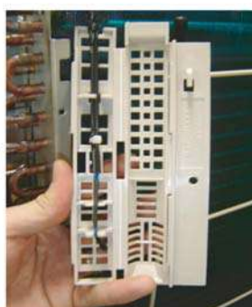
Open the THERMO HOLDER and remove the THERMISTOR.
