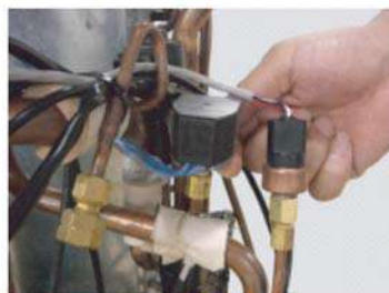
Remove the SOLENOID COIL.
