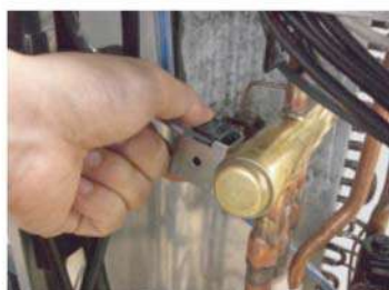
Remove the SOLENOID COIL.
