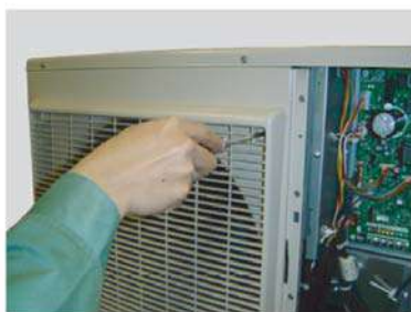
Remove the 4 mounting screws.
