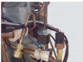
Remove the mounting screw.
